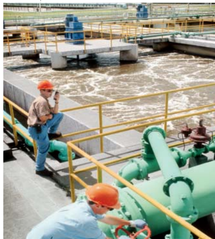
Figure 9 Bubbles pumped into sewage provide oxygen to bacteria that break down organic molecules. Next, anaerobic bacteria break sewage down further and generate methane, which is used to power the plant.
